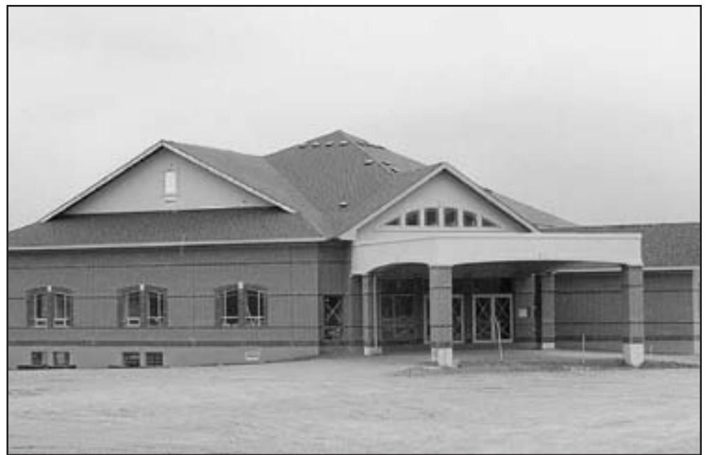
Caledon Hills Fellowship Baptist Church has opened its doors of its new building on Airport Road. the congregation is hosting its annual hayride this weekend.
